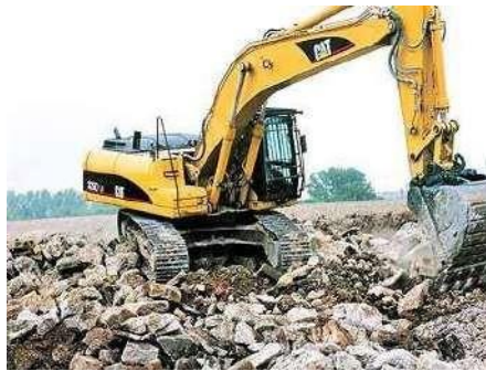
Fig. New Power Shovel
