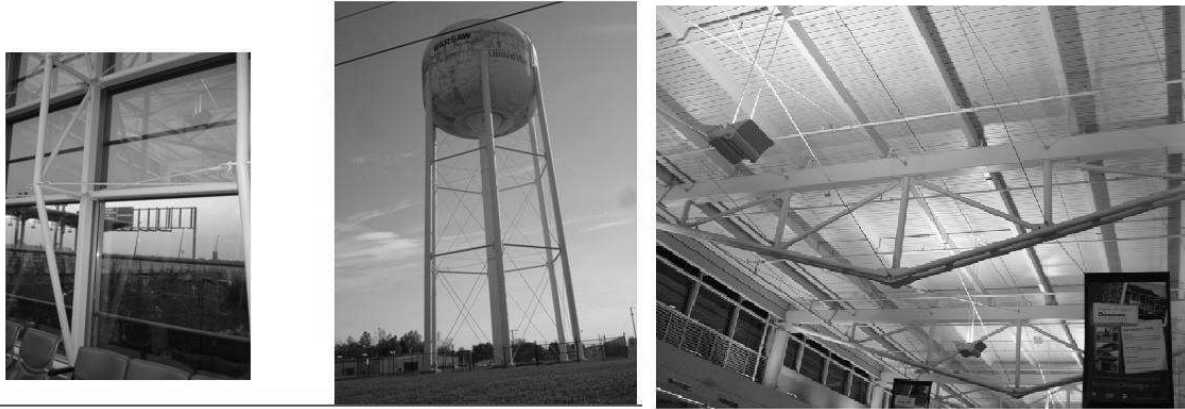
Tie Rods in Structures
